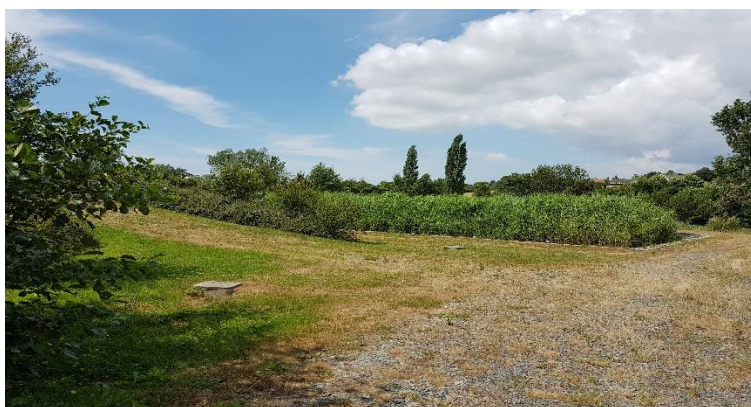
Station d'épuration de Quetteville-sur-S./Contrières
